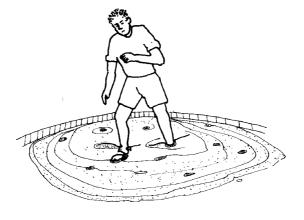
This is the more common way of mixing for a small-scale production.  $4 \text{ m}^3$  /day/man
